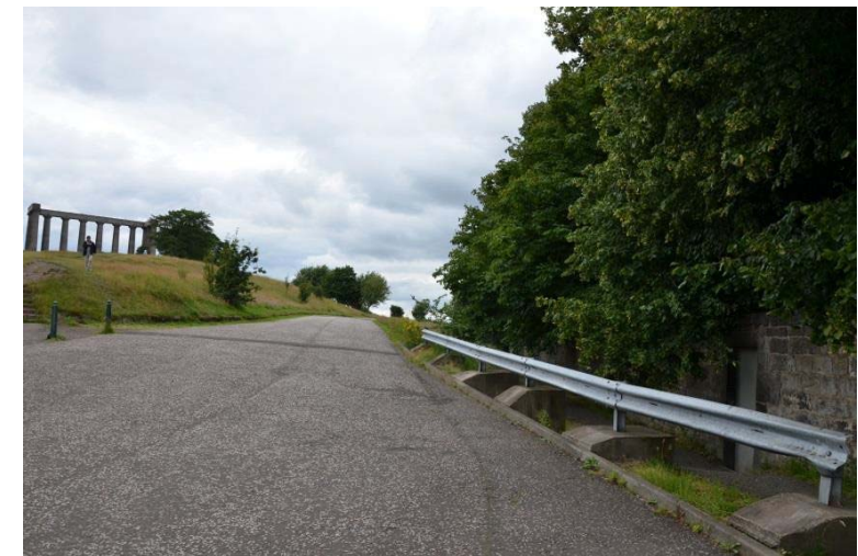
Crash Barrier at Calton Hill Drive / Regent Gardens Path
